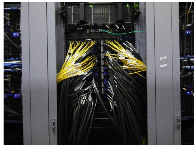
Rear view of Infiniband switch and cables (yellow=fibre, black=copper)
